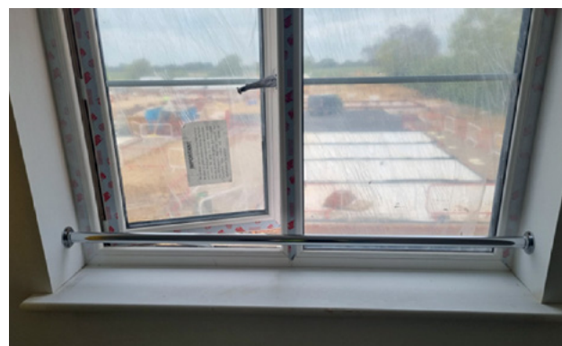
Figure 1: Example of a Part O compliant guard rail
